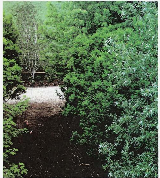
Bottom: Installing a 6ft evergreen hedge is all in a days work for the Majestic planting team
